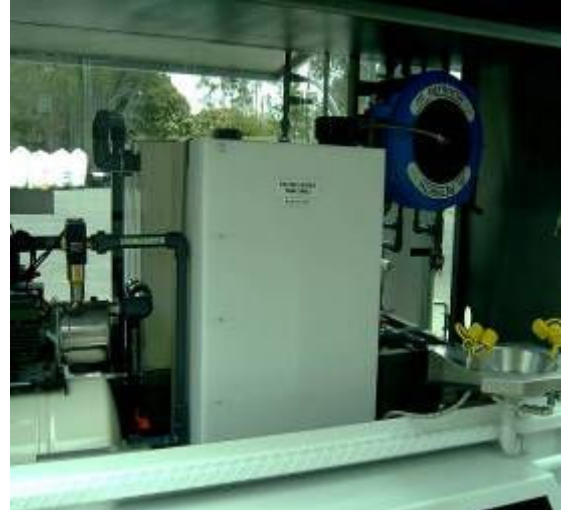
Photo 8— Potable Water Storage Tank
