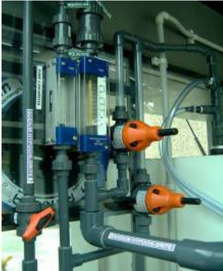
Photo 4 – Flow Indicators and Pressure Relief Valves
