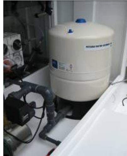
Photo 13— Potable Water Pressure Vessel
