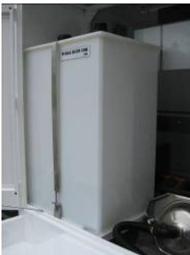
Photo 14 - Potable Water Storage Tank
