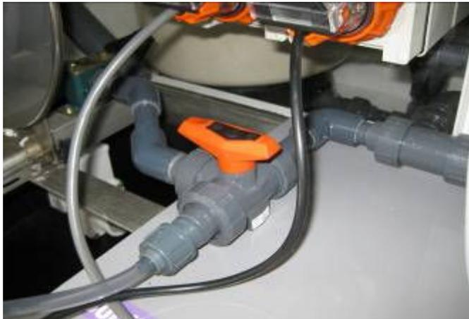
Photo 7—Manual 3-Way Valve (Selection of Chemical or Potable Water)
