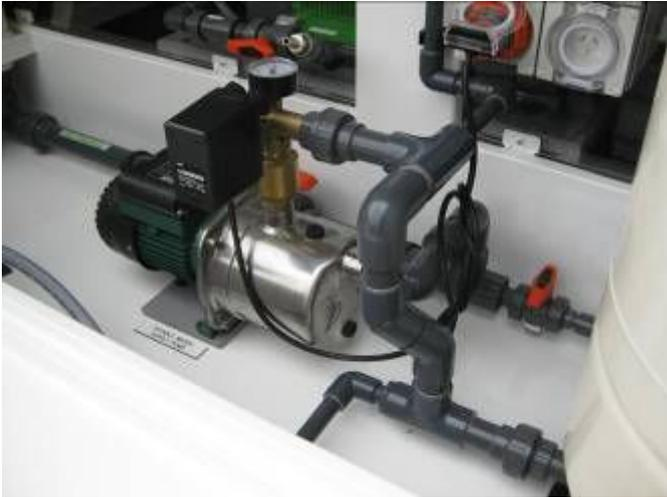
Photo 12 – Potable Water Delivery Pump
